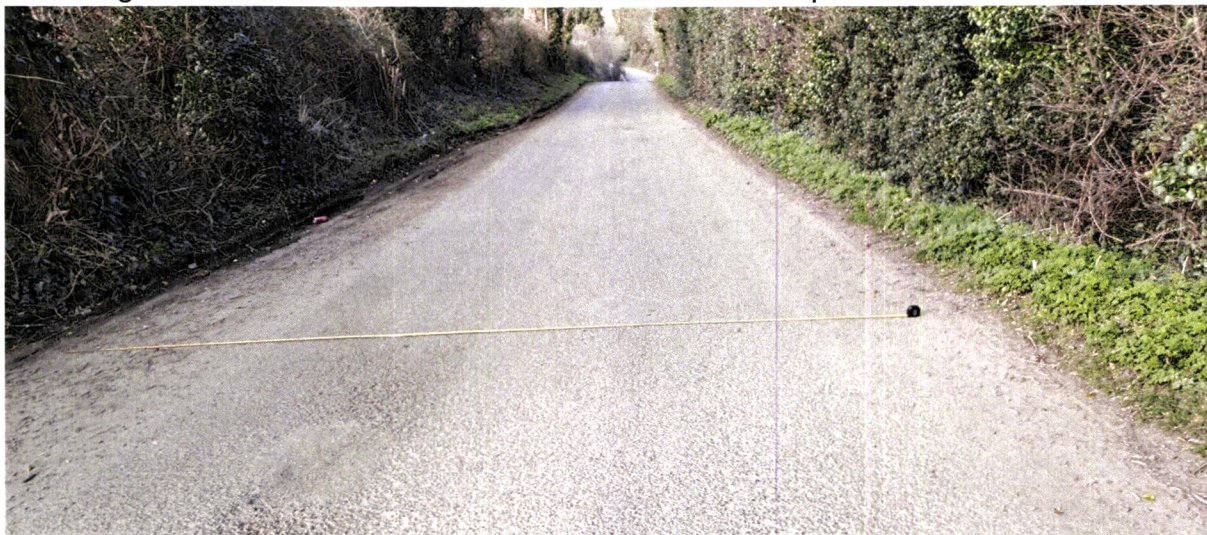
Barnaslingan Lane is measured to exceed 4m in width. Note the tape shown exceeds 5m in width.
